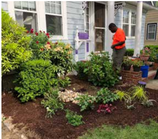
The Woonasquatucket River Watershed Council worked with homeowners in Elmhurst for stormwater retrofits, including redirecting roof downspouts away from the road and toward existing landscaping, installation of permeable pavers in place of walkways, and construction of rain gardens.
